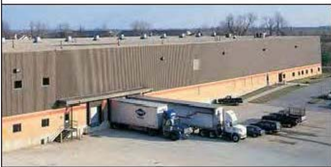
Link-Belt Parts Distribution Center
